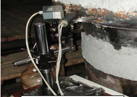
During weld joint check
